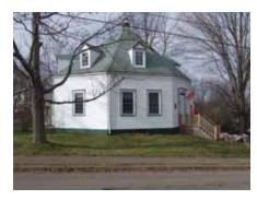
Undertaking a successful large-scale addition to a historic place is challenging. For certain buildings with a distinctive form it may be almost impossible. The Fraser Octagon House in Tatamagouch, NS is a one-and-a-half storey wood frame structure built to a near octagonal plan form. A large addition to this unusual character-defining form would be very challenging.
