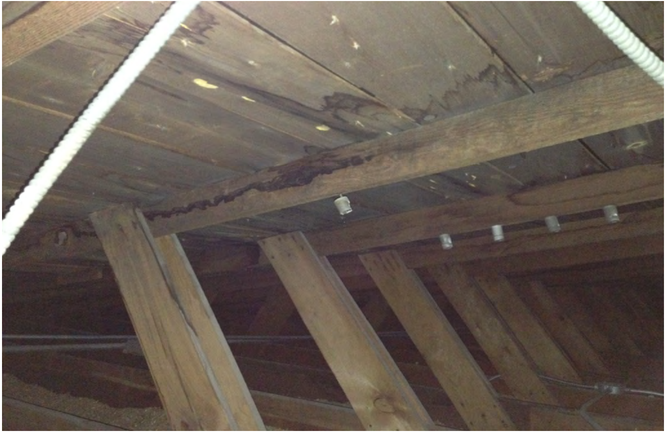
Photo 14 - Roof trusses with shiplap boards.
