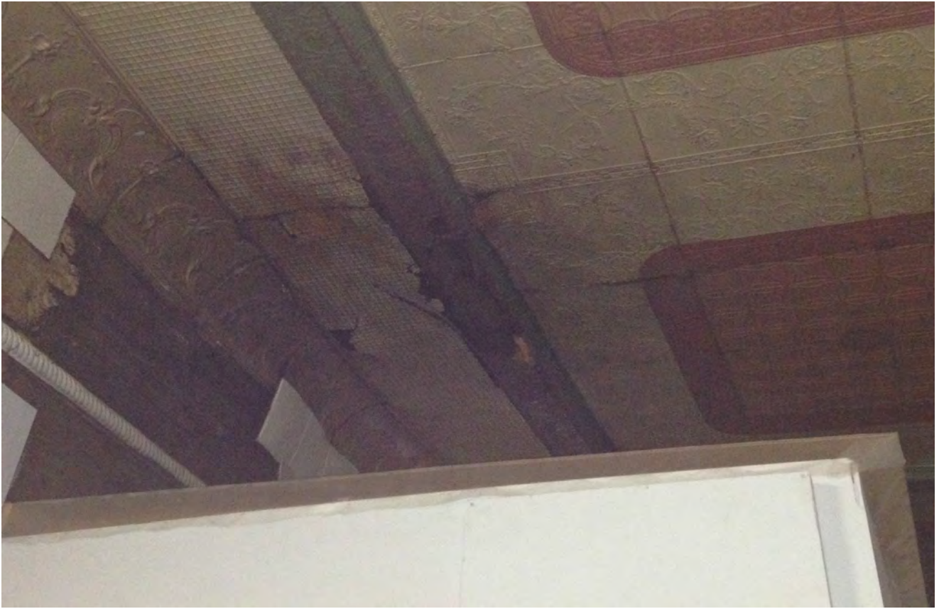
Photo 7 - Damaged tin ceiling at underside of roof trusses.
