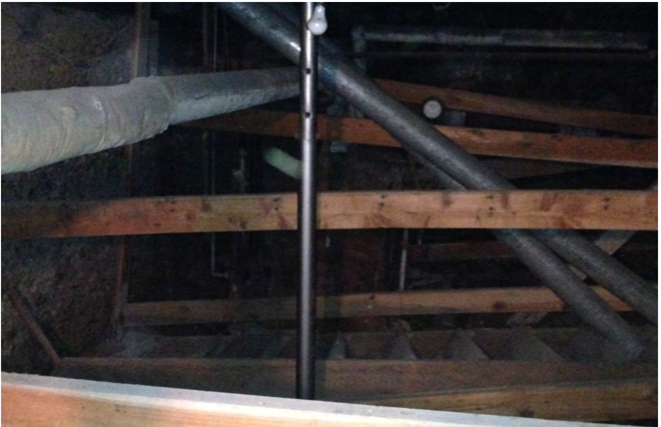
Photo 11 -Bracing in crawl space.
