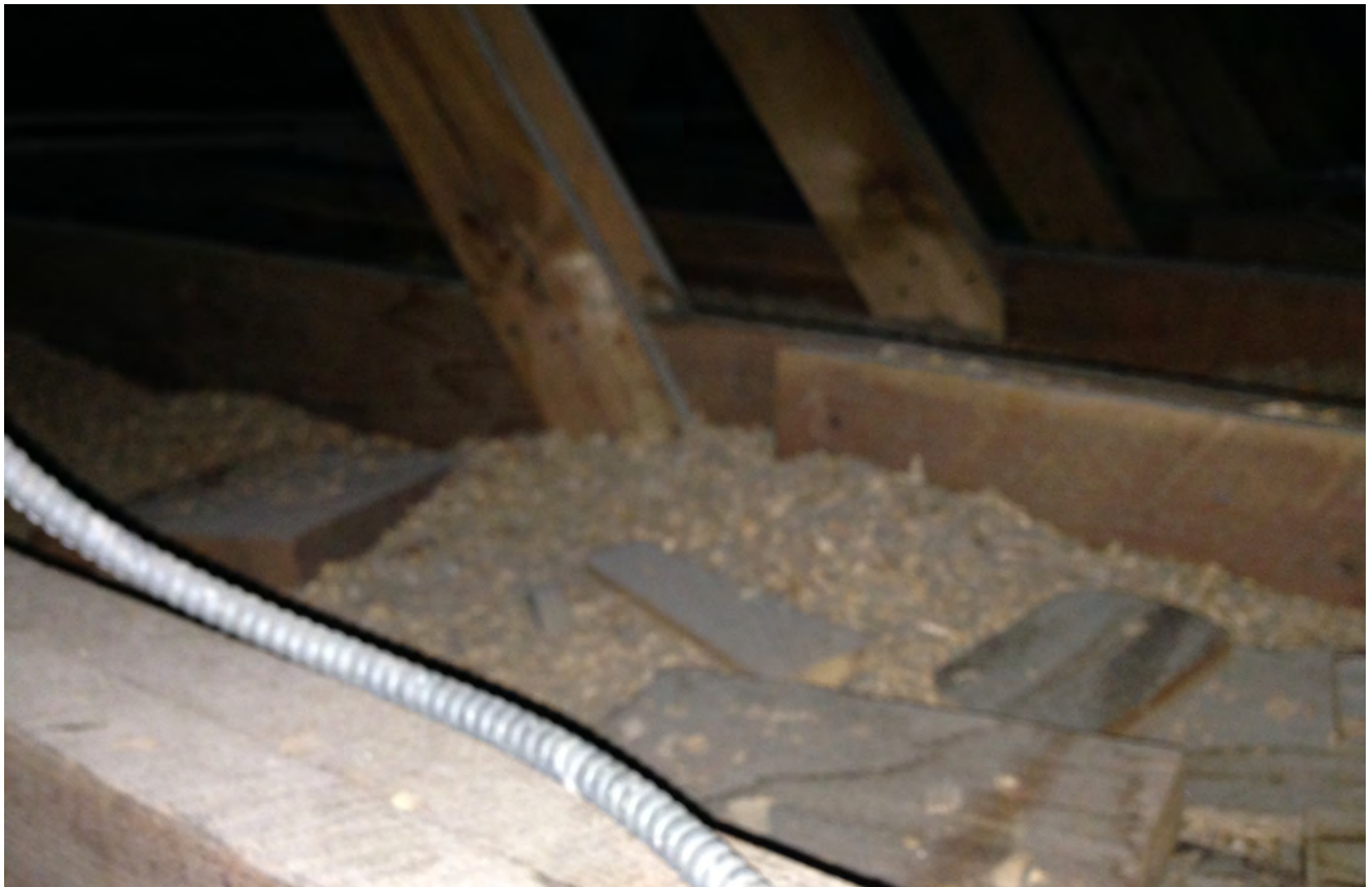
Photo 15 - Woodchip insulation between trusses.
