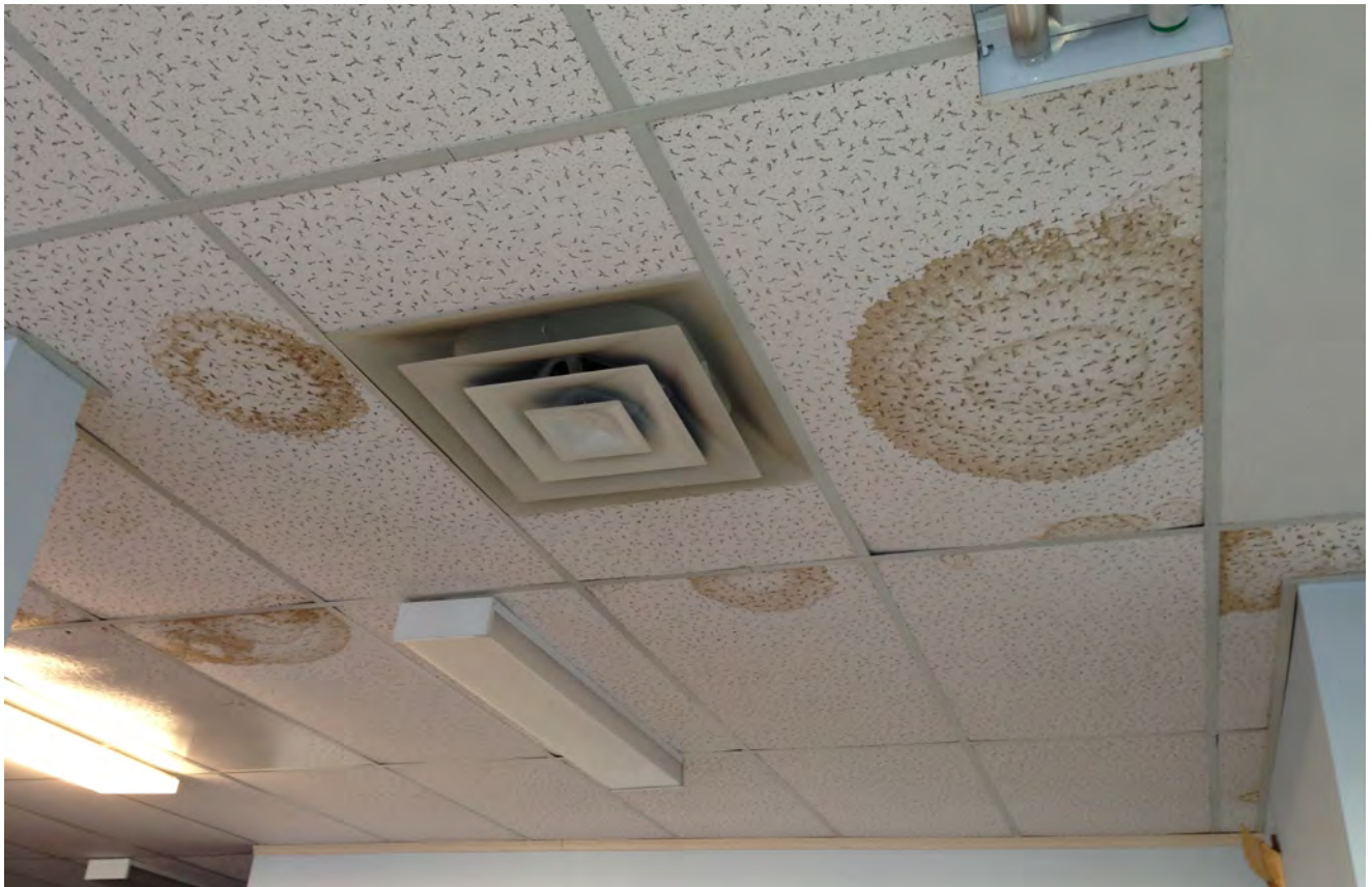
Photo 6 - Suspended ceiling below mezzanine
