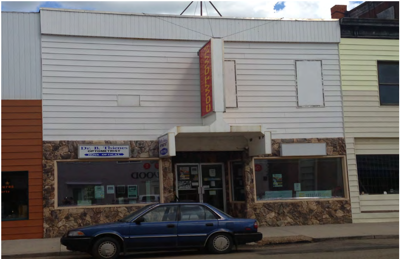
Photo 1 - Front (West) Elevation
