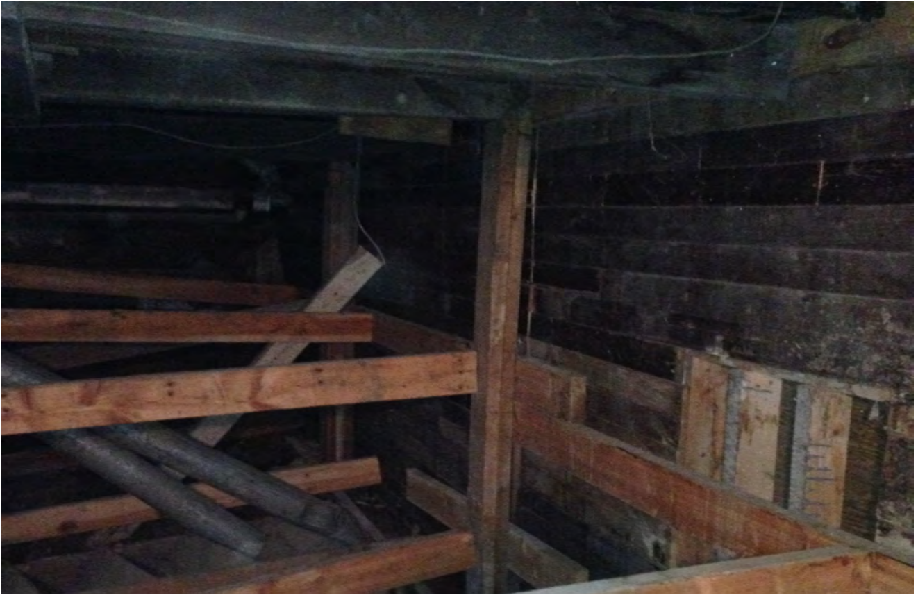
Photo 12 - Bracing in crawl space.
