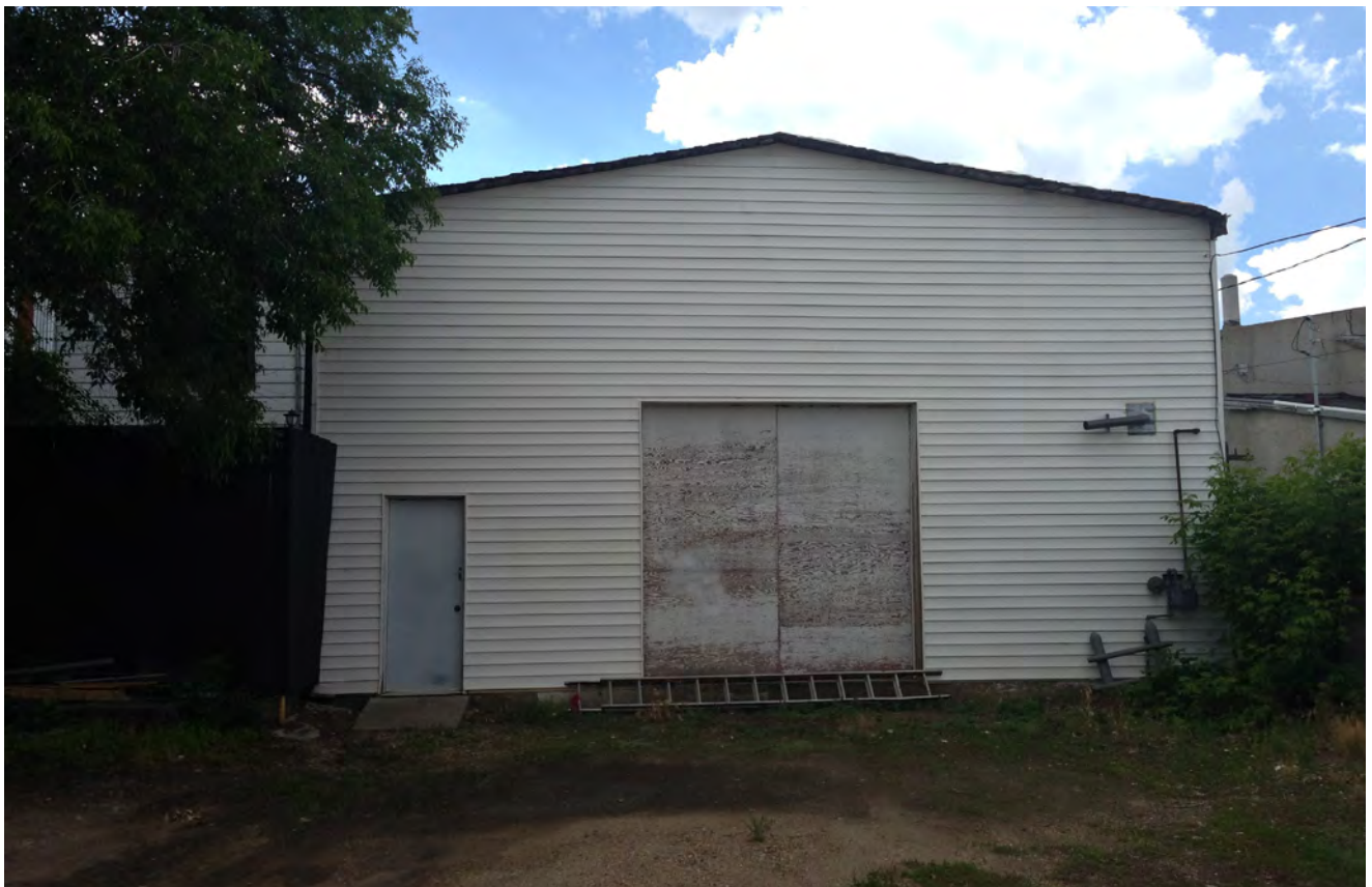
Photo 2 - Back (East) Elevation
