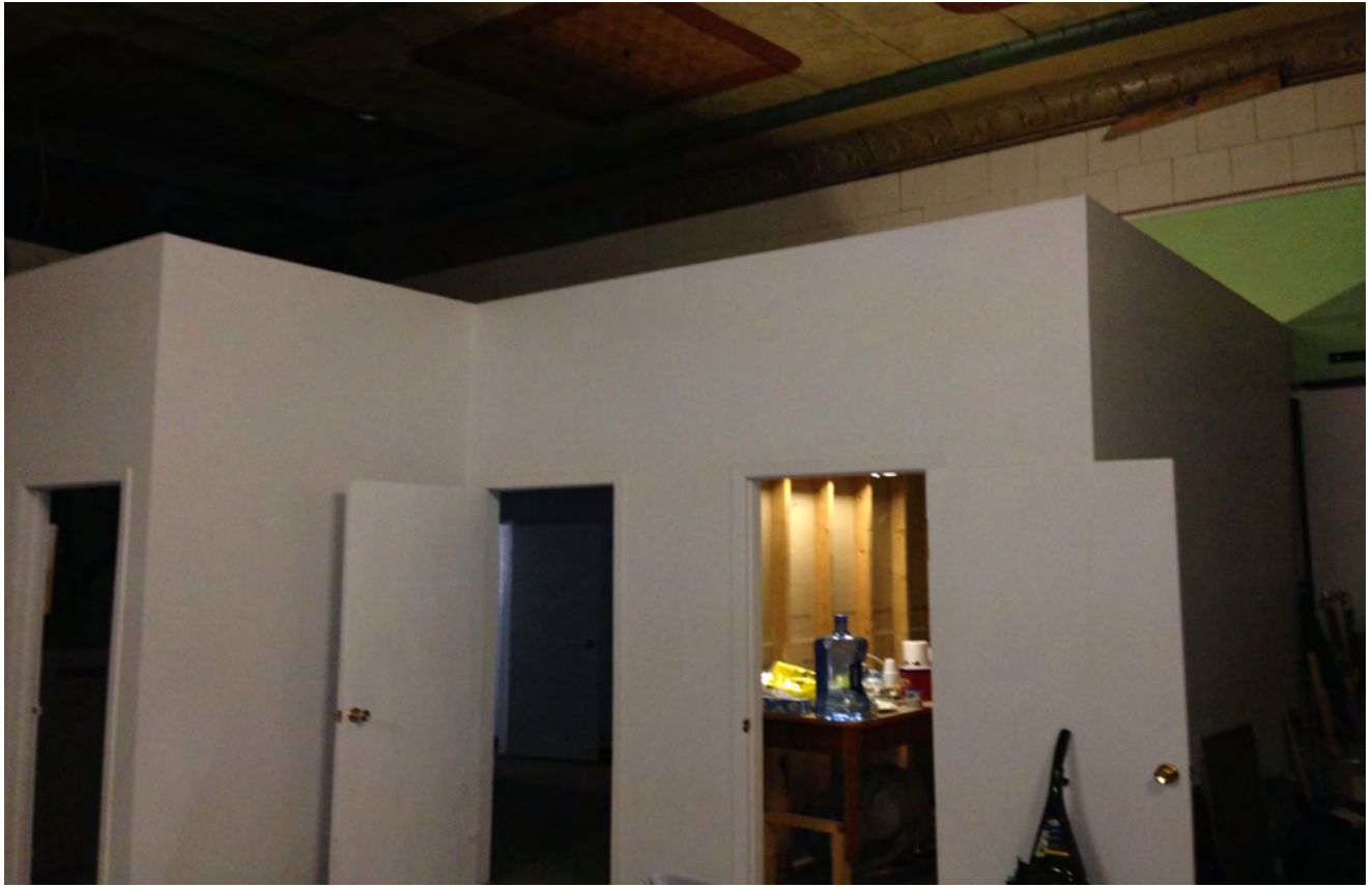
Photo 5 - Interior partitions and ceiling (built as structure within structure)
