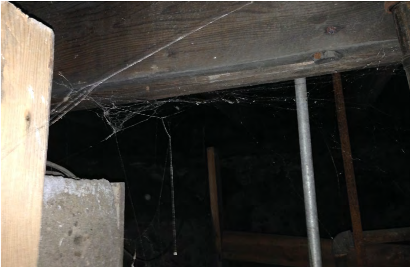
Photo 13 - Beam supported by temporary steel shoring post.
