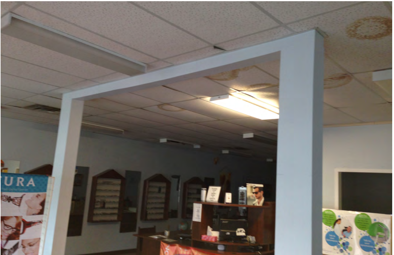
Photo 8 - Mezzanine supported on two posts
