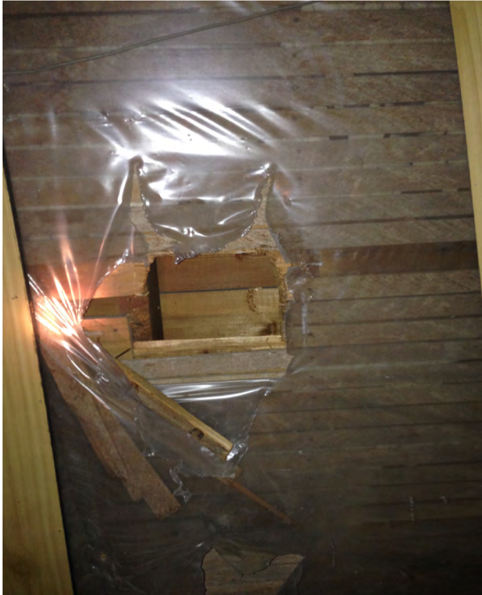
Photo 9 - Exploration hole in South wall
