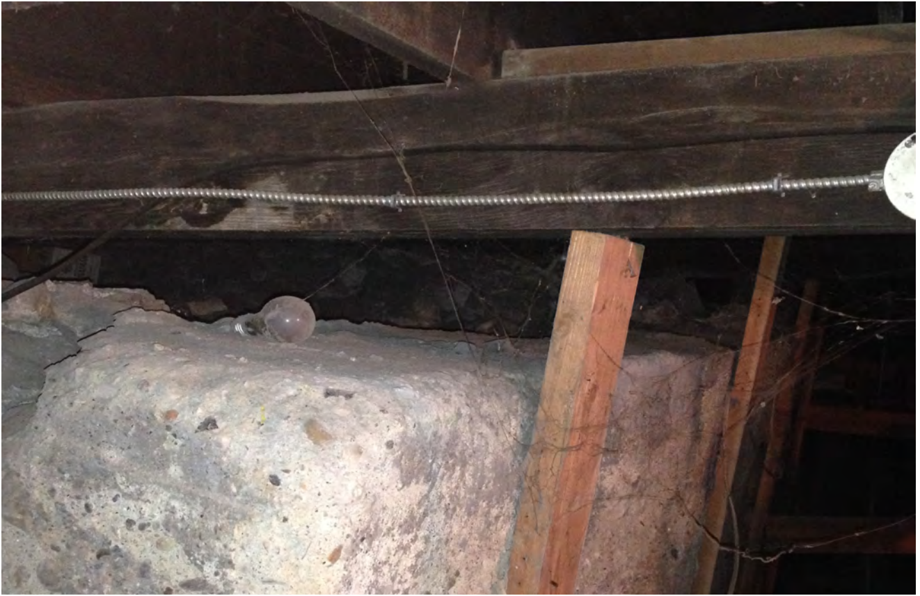
Photo 10 -Mass concrete retaining wall separating crawl space.
