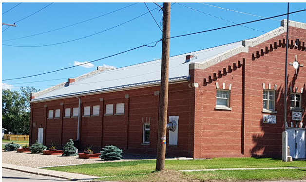
CiB installed a Colorado Blue Spruce 'Living Fence' at the Maple Creek Armoury, a designated heritage building. Work has progressed with the addition of raised flower beds.
