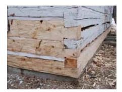
Deteriorated logs at the John Walter Historic Site in Edmonton were replaced in kind with hewn logs that used the originals as templates to reproduce tooling marks on visible surfaces. On close inspection, this distinguishes the new materials if the logs are separated in the future.
