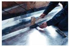
When restoring the former post office in Dawson, YK, the metal roofing surface, which was too deteriorated to repair, was replaced in kind. Physical evidence from the restoration period was used as a model to reproduce the characteristic standing seam detail.
